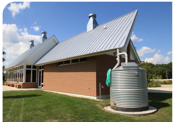
Cisterns minimize discharge of roof runoff to the closed drainage system, and allow water reuse for irrigation or other functions
