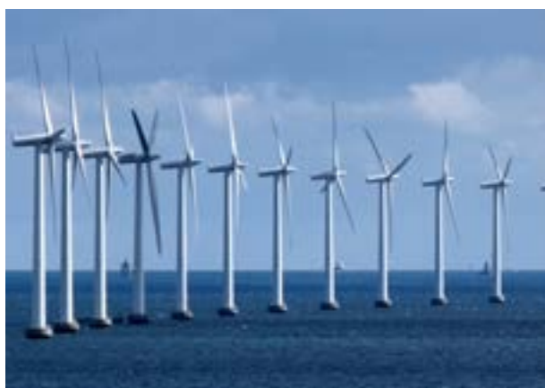
Middelgrunden Offshore Wind Farm
