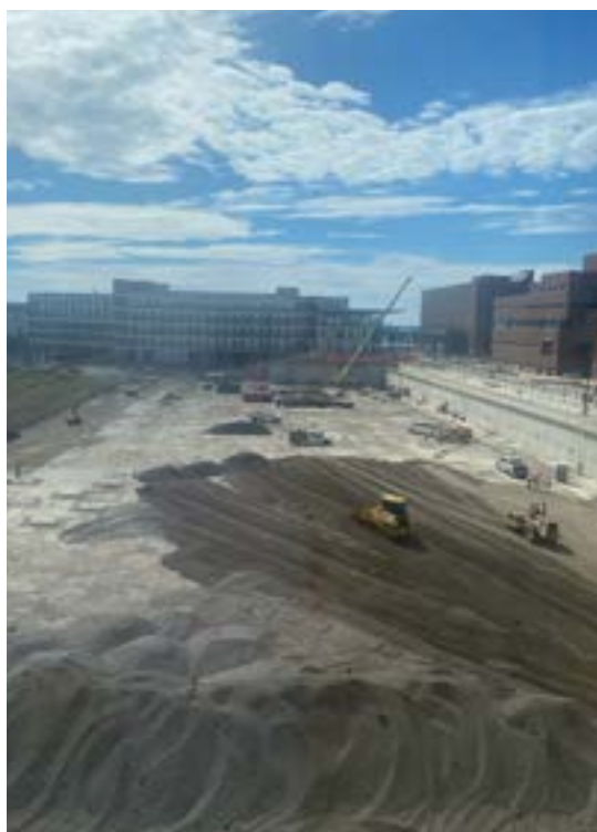
Crews move materials into the quad.
