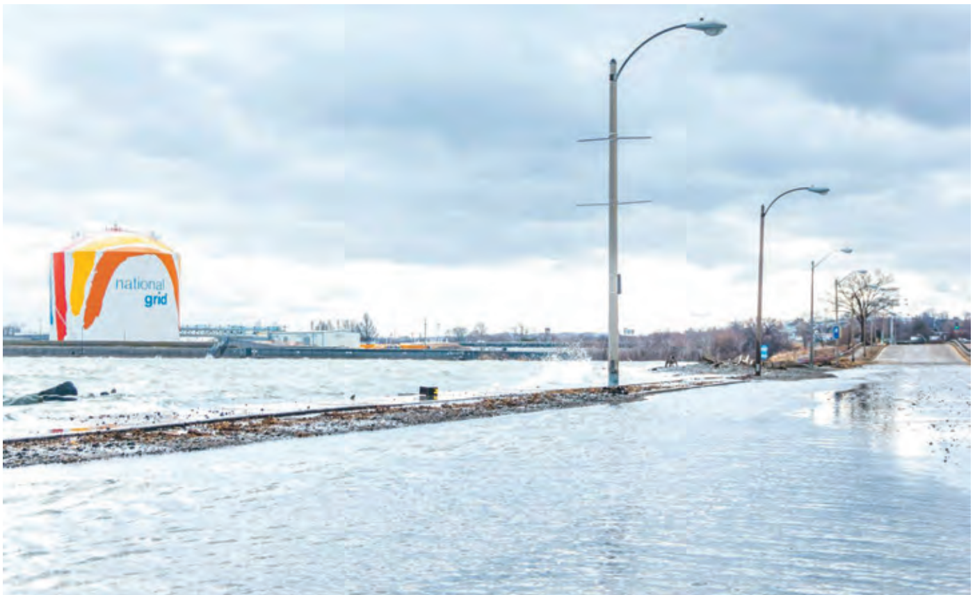
Flooding on Morrissey Blvd in Dorchester, Boston. March 2018.
